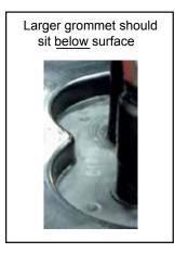
3/4-Inch grommet should sit slightly below flush with surface
